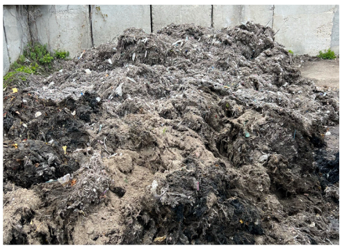
Pile of about 30 yards of wipes and assorted personal care items (q-tips, women's feminine products, etc.) that were flushed down toilets that had to be cleaned out of a digester.
